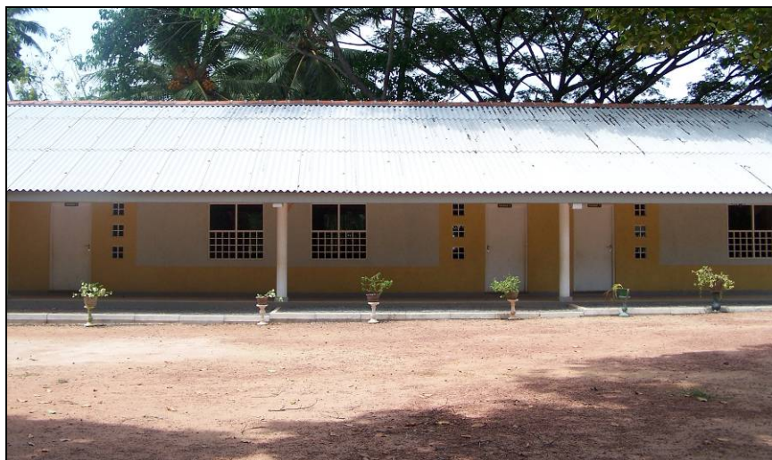
First block of classrooms built in 2007
